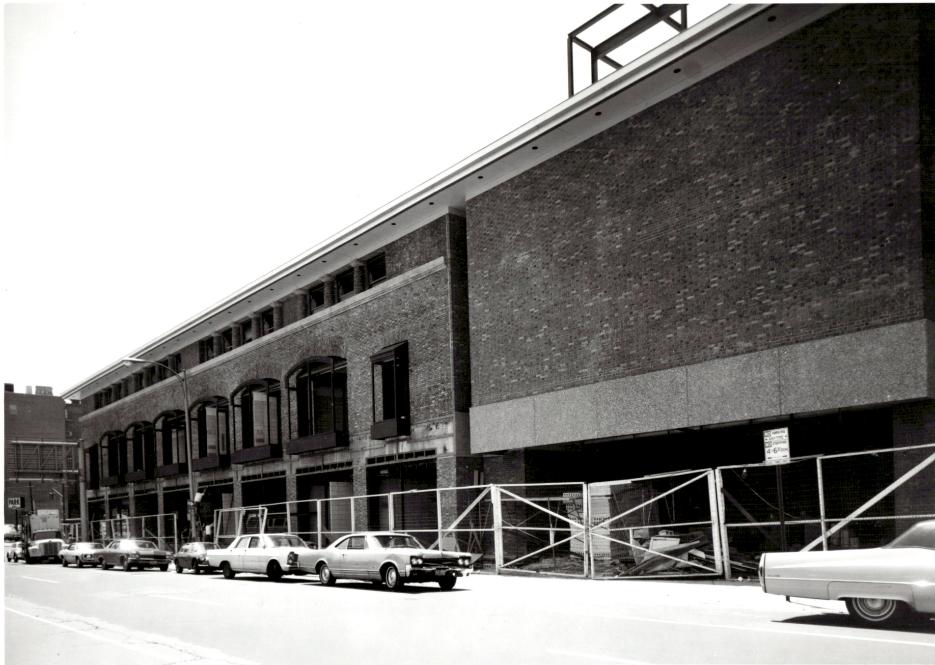
ACADEMIC CENTER UNIVERSITY OF BALTIMORE ROY KIRBY & SONS, INC., CONTRACTOR FISHER, NES, CAMPBELL & PARTNERS, ARCHITECTS GENERAL VIEW LOOKING SOUTHWEST JUNE 1, 1971
