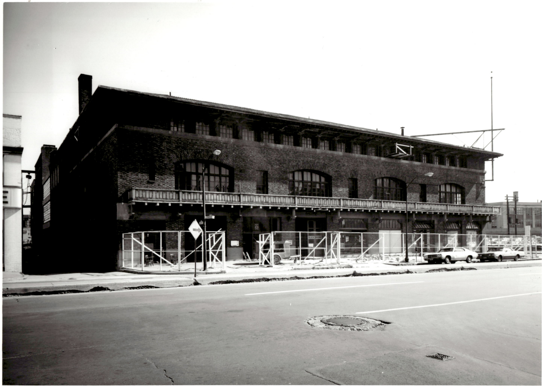
ACADEMIC CENTER UNIVERSITY OF BALTIMORE ROY KIRBY & SONS, INC., CONTRACTOR FISHER, NES, CAMPBELL & PARTNERS, ARCHITECTS GENERAL VIEW LOOKING NORTHEAST AUGUST 4, 1970
