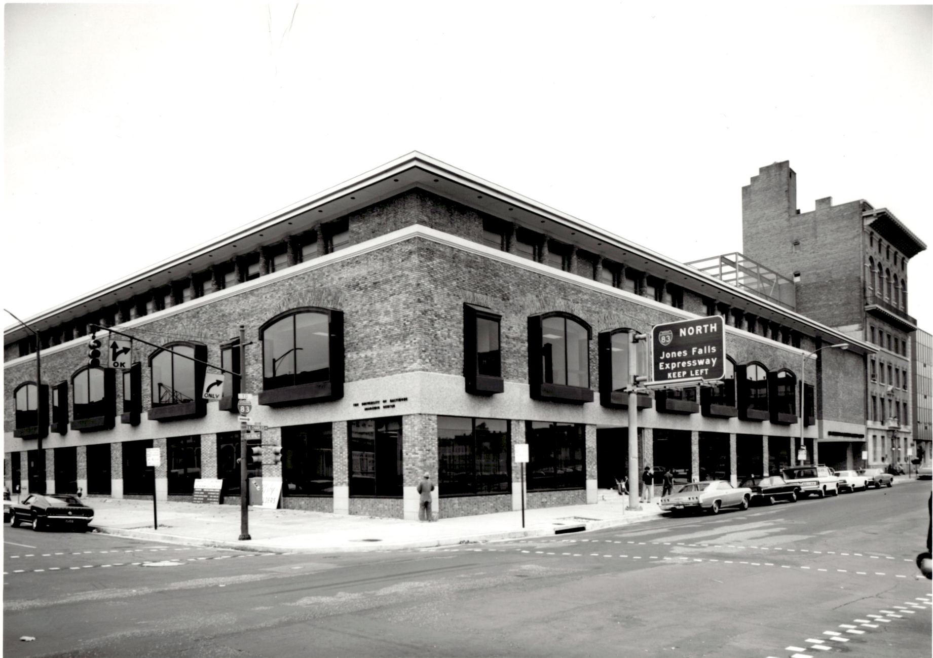
ACADEMIC CENTER UNIVERSITY OF BALTIMORE ROY KIRBY & SONS, INC., CONTRACTOR FISHER, NES, CAMPBELL & PARTNERS, ARCHITECTS GENERAL VIEW LOOKING NORTHWEST OCTOBER 1, 1971
