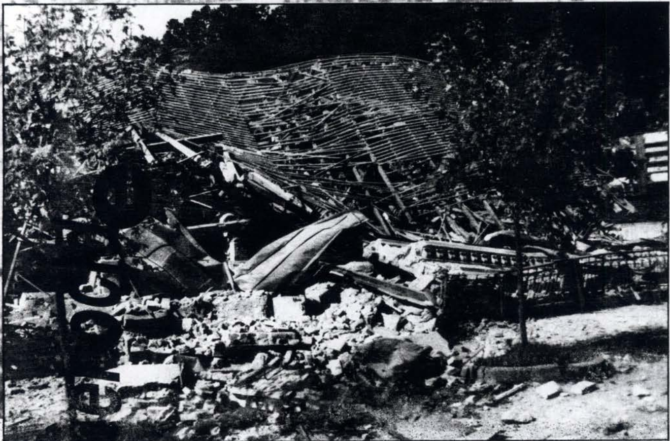
A nd in this demolished house, at Topusko, there was a museum with a documentation about the Fascist crimes against the Serbian people committed in the Second World War .
