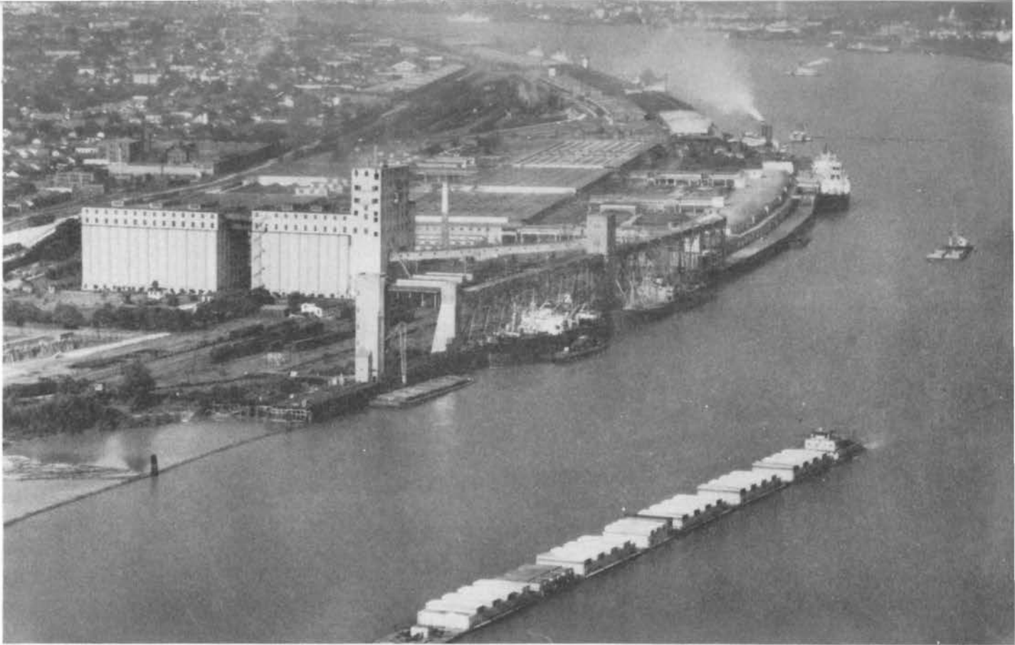
New Orleans Public Grain Elevator. This elevator is equipped to unload grain from, or load into, ocean-going vessels, barges or railroad cars. It is also well equipped for sacking grain and has a storage capacity of 2,622,000 bushels.
