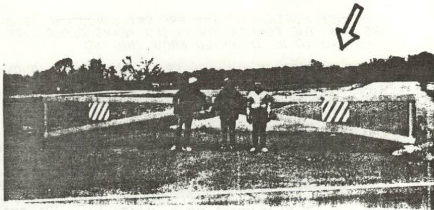
BARRIER GATE AT SHAW SITE [ARROW]
