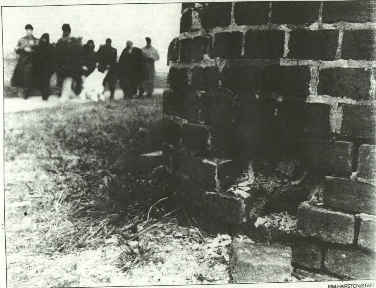
Bricks have fallen from this interior wall at Fort McHenry, which withstood British shells in 1814. American Legion is raising money for repairs to the monument.
