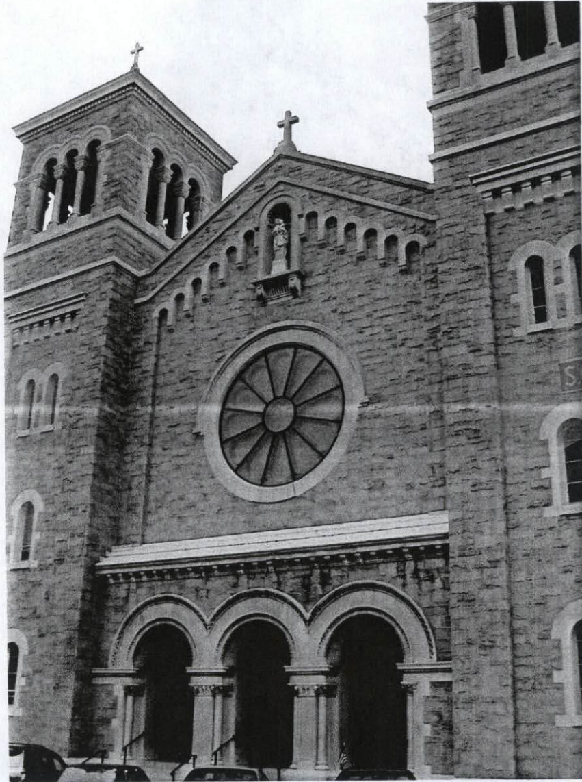
Holy Rosary Church is located on Ann Street in Baltimore, Maryland.
